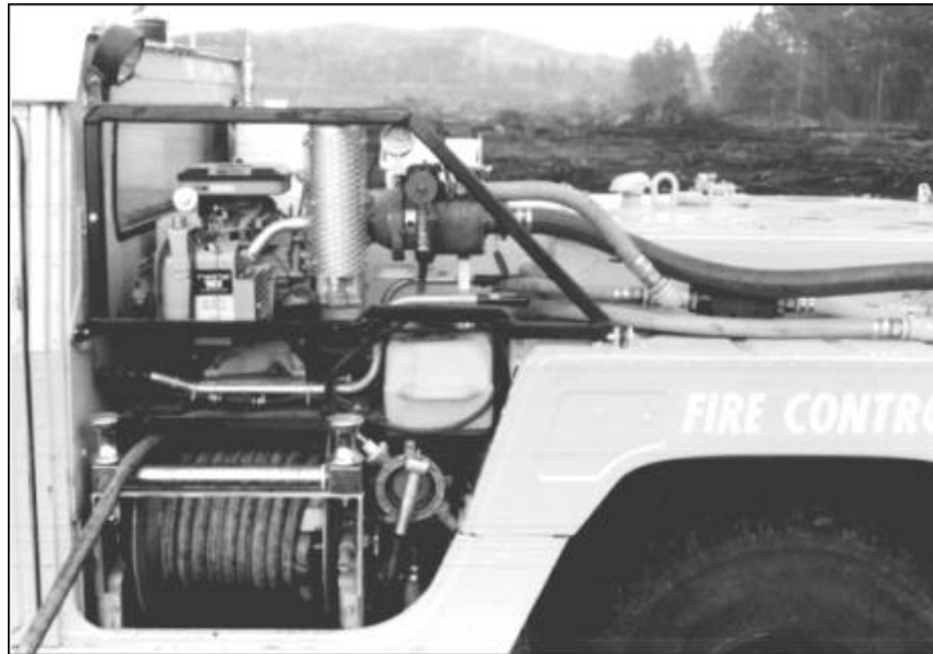
Figure 3 - The pump and left hose reel were mounted in the rear passenger area.
